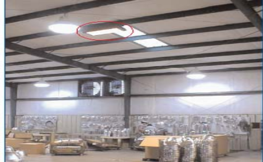
A radiant heating system will feel warm even though the surrounding air temperature is significantly lower.
