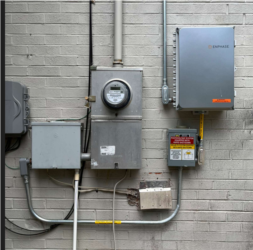
Example 3: Post installation picture of meter socket and newly installed PV AC disconnect
